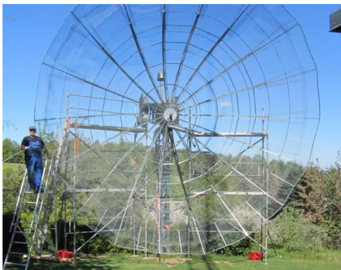
DL6SH and dish during 2020 refurbishment
