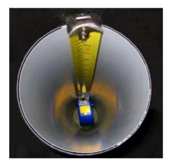
The following picture shows the construction of a rope winding drum, made from some M8 studded rod, two CD's and a short length of plastic conduit.
