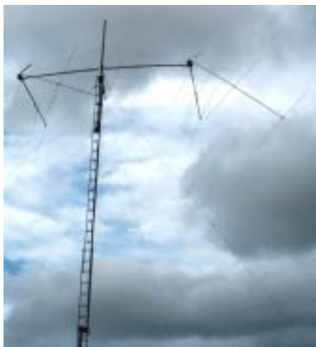
ZL2DX Six Metre Yagis after wwindstorm.
