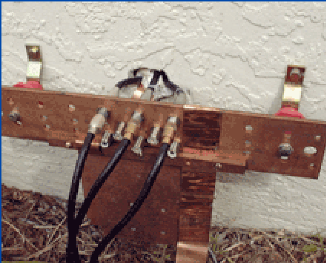
Single point ground outside of house (point of entry)
