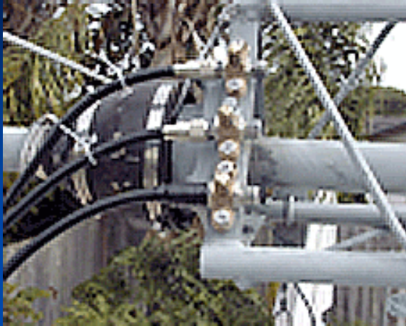
Coax shields grounded at top of tower
