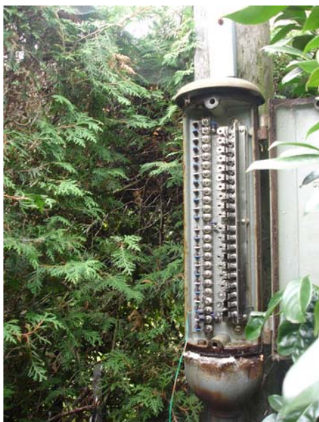
Figure 10: signal injection at the transition pole
